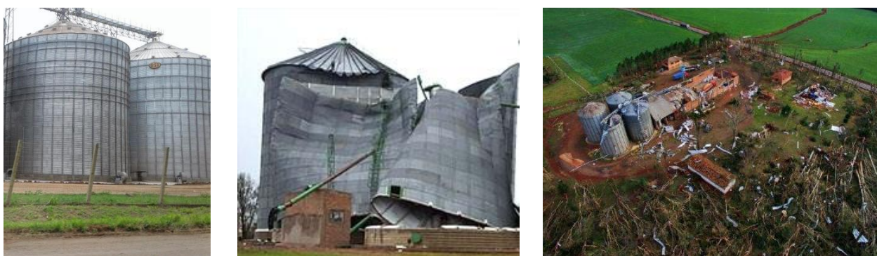
Figure 1. Typical external configuration of flat silos and pictures showing silos after accidents caused by the wind.
