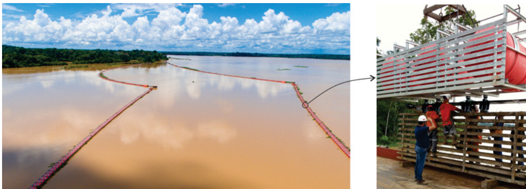
Figure 1. Log boom line in the Madeira river (left) and a log boom module (right)
